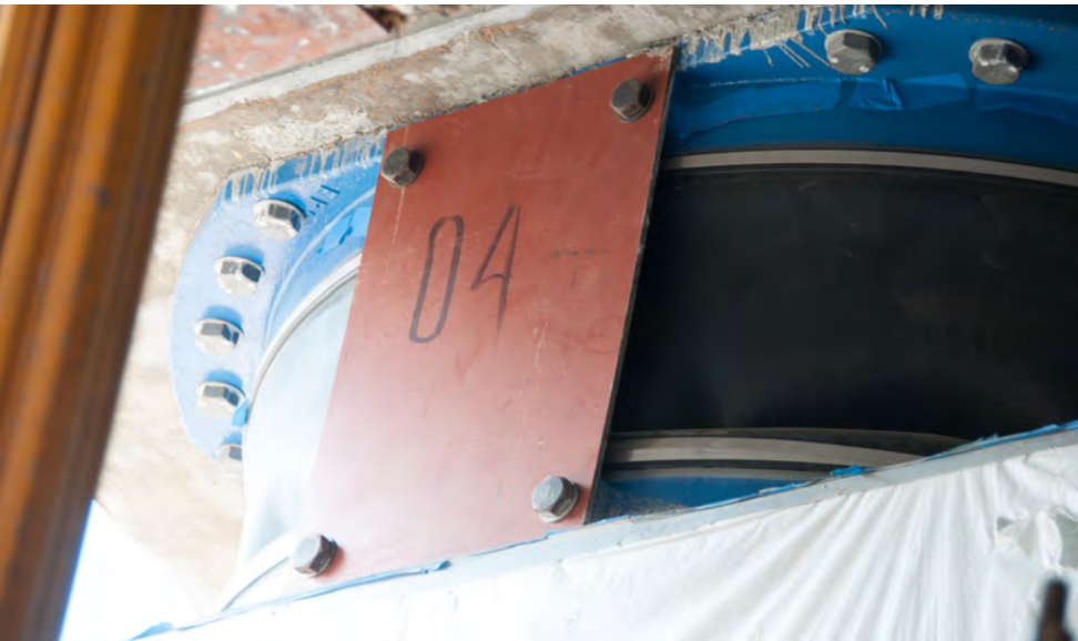
▶ This is one of the seismic isolators. The red-metal plate prevents any movement during construction and will be removed when the shoring towers are removed.
